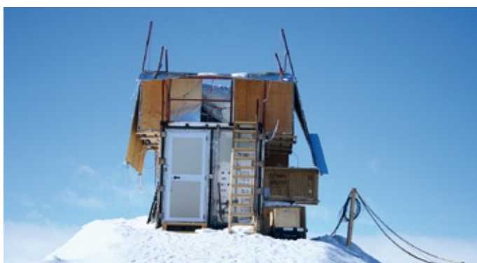
Colonisation 2041, Shelter Brain, abri d'un instrument astronomique du programme BRAIN à Concordia / Shelter of the BRAIN program astronomical instrument at Concordia
